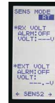
Set audible alarms to alert you to low battery voltage or high temps.
